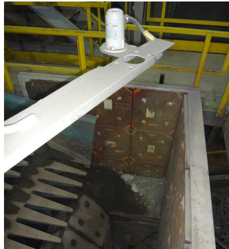
Crusher level measurement with laser in the mining industry.
