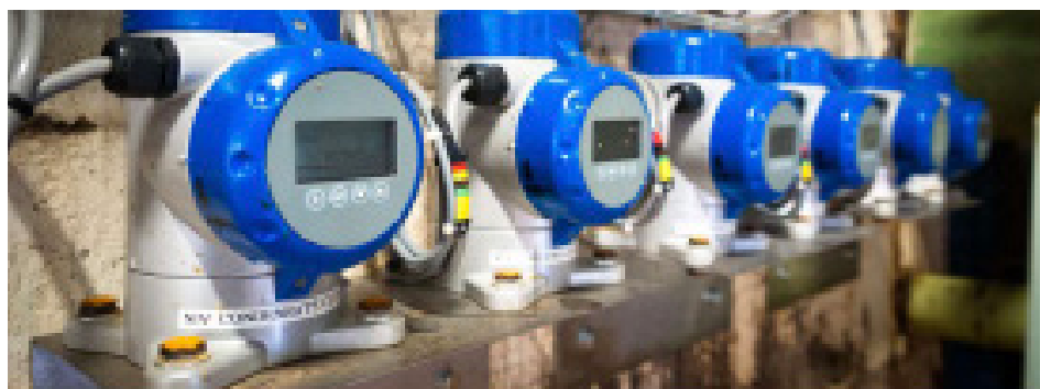
OPTIFLEX 7200 used for measuring cleaning water at a waste treatment plant.
